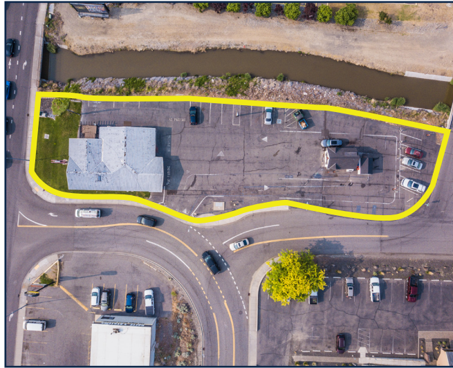
N Columbia Center Blvd. - Kennewick WA
